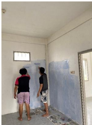
Gambar 5. Pengecatan central education
